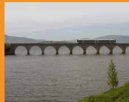
Railway bridge. Arija
